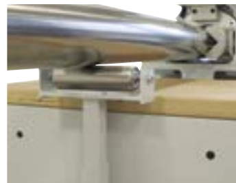
Roller pipe support
